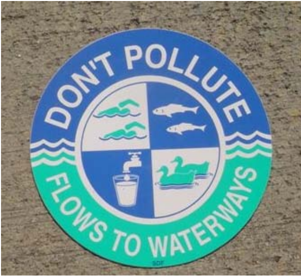
Typical Storm Drain Marker
