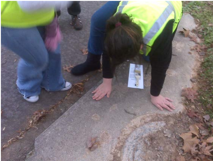
Volunteers install a marker on catch basin in Brookside Subdivision.
