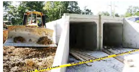
Before and after of a culvert replacement on Beaverdale Rd. where Whitfield County saved approximately $300,00 by utilizing its on public works department rather than a contractor
